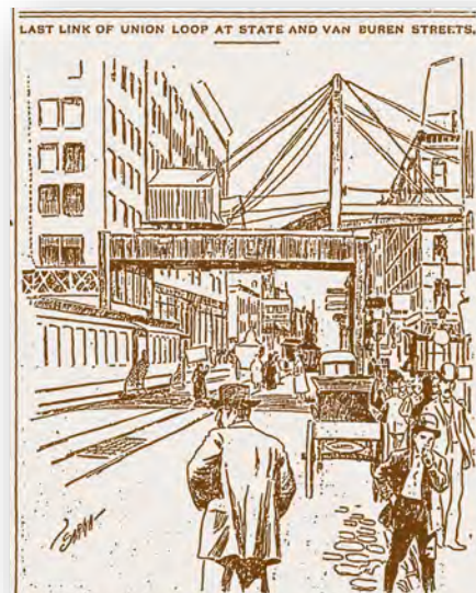
"Last Link of Union Loop at State and Van Buren Street" illustration by Charles Sarka, Chicago Record , January 1, 1897. The caption read in part: "At State and Van Buren streets the contractors for the Union Elevated loop have erected the largest single span on the system. It measures more than 100 feet, and a day and a half was taken in getting the iron in position."
