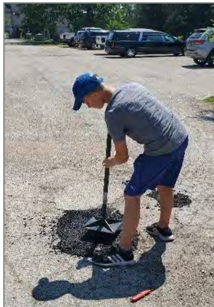
Connor Michalek, one of our younger volunteers, perfects his pothole patching skills.
