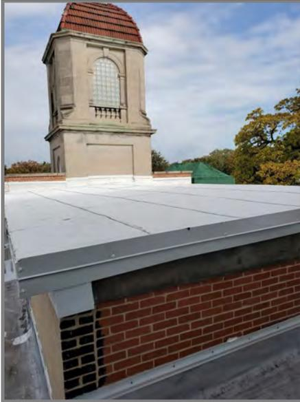
to donations from Friends of BNC members and supporters. As reported in previous newsletters, important repairs were made to several rooftop masonry walls, including reconstruction of parapet walls connecting to the northside bell tower.
