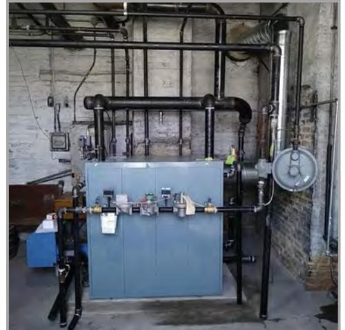
*Workers from Williams Stoker removed BNC's old boiler located in the lower level of the crematorium/columbarium building (left) and replaced it with a new high-efficiency unit.
