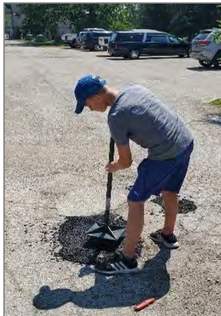
Connor Michalek, one of our younger volunteers, perfects his pothole patching skills.
